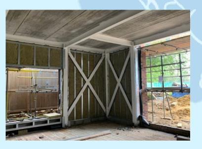
Internal ground floor, showing the steel frame, cement boards and the start of insulation.
