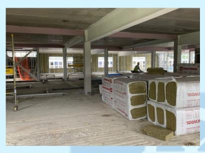
A picture of the ground floor showing the fireproofing of steelwork and storage of insulation boards.
